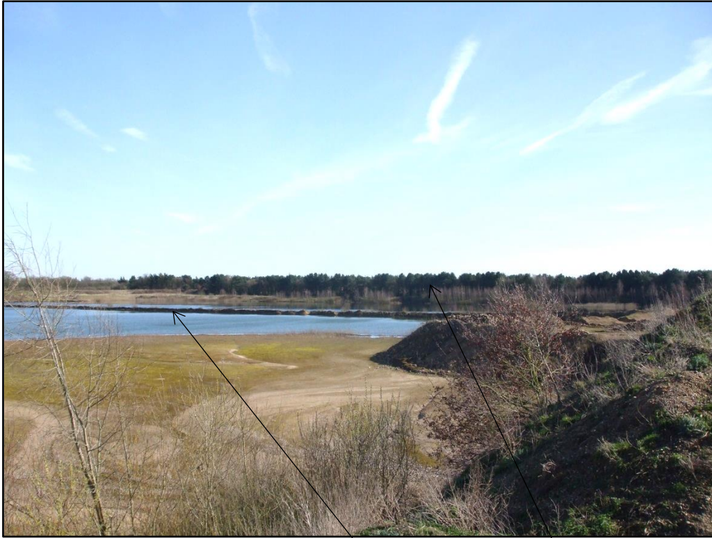
Photograph 1 – Conveyor route causeway and advance planting along southern boundary
