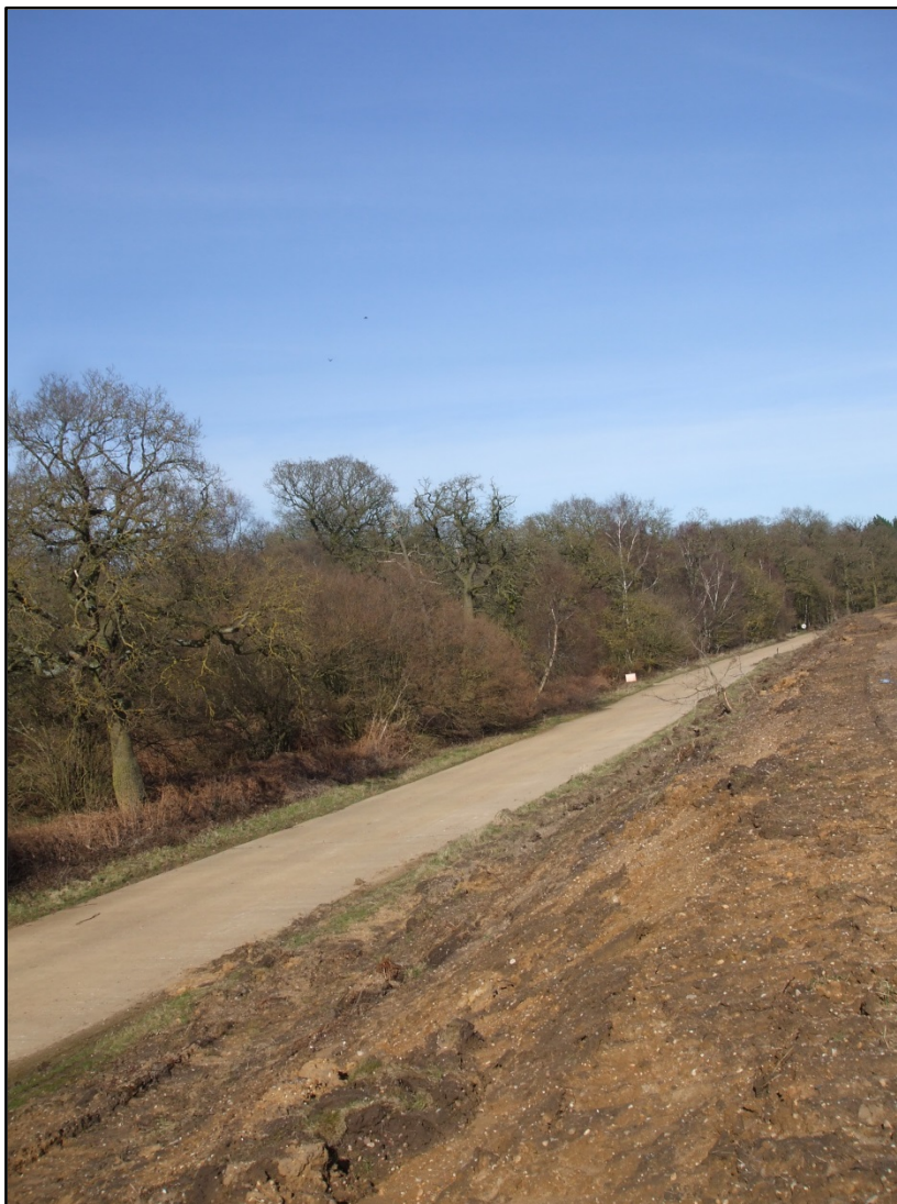
Photograph 2 – Concrete haul road
